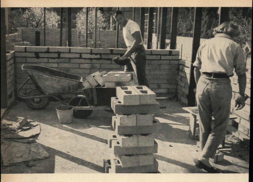
For an owner-built house, concrete brick was a wise choice of material since it is thick enough to require no inside wall construction, and because the small units are relatively easy to handle. When they were delivered, they were set in piles near the spots where they were to be used—a bit of foresight which saved the Booths both time and labor
