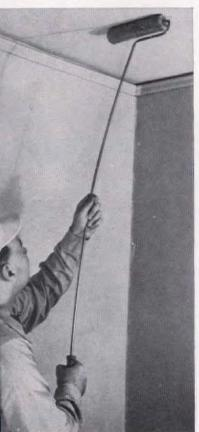
A long-handled roller, or a regular roller with a long handle improvised and fastened securely to the short handle, will do away with much of the ladder or scaffold work on ceilings and high parts of walls. It will reach behind radiators too. Painting or varnishing floors, the same long-handled roller saves backaches
