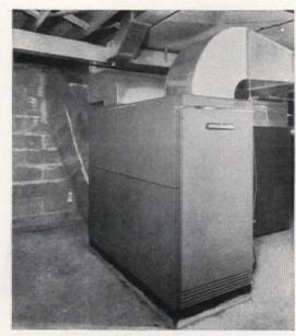
HEAT PUMP keeps you cool in summer, warm in winter. It runs on same principle as refrigerators. In winter, it draws heat from outside air to warm house. In summer it does the reversedraws off heat from air in the house. Automatic, it needs only electrical connections and ducts
