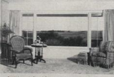
rior weather-tightness—because Silentite double hung wood windows have the famous Curtis "floating" weather-strips. Here, Silentites are either side of a Curtis picture window. used on
