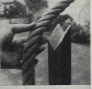
Make a 45° "V" cut at top of each post for rope. Rope can be held in place with strips of metal 34" wide or with regular pipe supports. Top end of rope may be attached to wood fence around roof or to top platform
