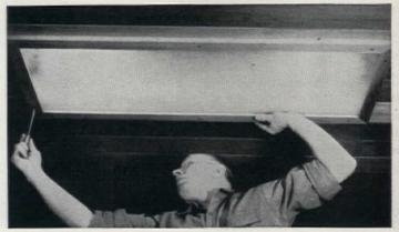
Frame two sides and one end of recess with ordinary 1 x 2 lumber, rabbeted to hold the glass securely. Slide glass into place and attach other end of frame
