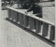
4" x 4" top support is 32" long. Cot 1" notch tapering to 0° to keep brace from slipping. Brace is 33" long and fits at 45°. Fasten support to post with U-shaped strap iron, or to wall studding with two metal straps
