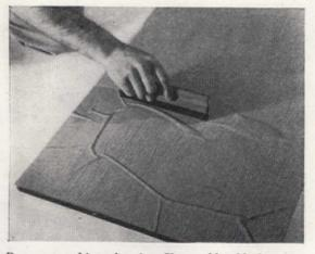
Proper smoothing takes time. Use a rubber block or squeegee to go over the surface-first lightly, then firmly. Then wipe surface with damp cloth. If any veneer hangs over, wait until cement is dry-then cut off excess with pencil wrapped in fine sandpaper
