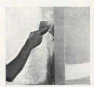
Additional coats of adhesive are applied over tape portion of bead so it is completely concealed. Don't move position of bead during this process
