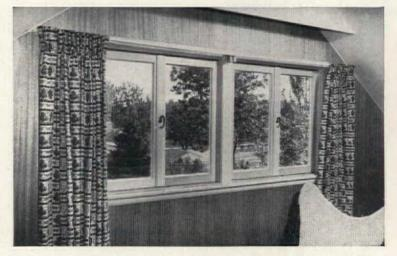
Here are close-ups of windows which do so much for rooms on page 57. One is a 5'6" x 4'6" sliding unit; the other a pair of sliding units combined to give a 3'6" x 7'6" opening. They cross-ventilate so well that this attic actually cools off faster than downstairs on hot days
