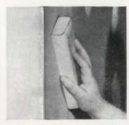
When the adhesive has become hard, remove the rough spots on the adhesive by sanding lightly. Wall surface is now ready for paint or wallpaper
