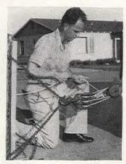
With one end of fence fastened to one corner post, fence stretcher is clamped to free end. As author hauls on tackle, his partner wires taut fence to other post
