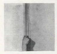
Apply adhesive to edges of the corner and then carefully bed the corner bead in place, working from top to bottom. Be sure that bead is vertical
