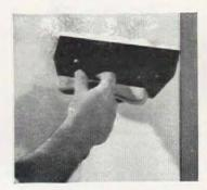
Use an extra-wide putty knife to feather out the adhesive to assure smooth joint between wall and bead. Remove adhesive from outside edge of bead
