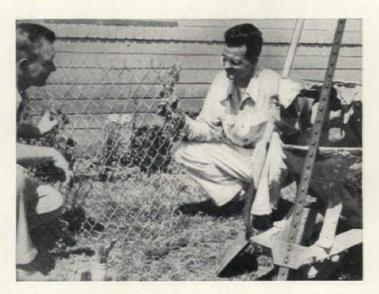
Neighbor Marc Pickrell, left (and in upper picture beside the twin gates), and brother-in-law Tom Clark look over the tools and materials used. Besides 36" chain-link fencing, they include posts, old bed rails, shovel, wheelbarrow, cement, coarse sand, wire-stretcher, electric drill, pliers, aluminum paint, brushes
