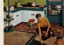
Here Mrs. Loock finds the center of the floor. Next, she'll spread Kentile Adhesive over half the floor before laying the tiles in place.
