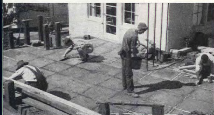
Progress—as the concrete is poured between the redwood strips. Note the four pipe supports for the future trumpet-vine trellis, the plant box, left open at the bottom for drainage, and, in the foreground, the top of the new, higher redwood retaining wall
