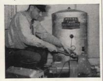
STEP 2. Installing water system. Myers home water systems are operated by electricity and completely automatic.
