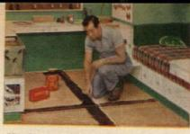
Handy Ken-Kit has complete instructions—all the tools you need. After the floor has been measured, chalk line is snapped. Next, Kentile Adhesive is spread.
