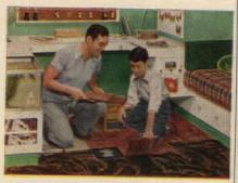
Tiles go down one at a time over first half, then Kentile Adhesive is spread and tiles set in remaining area. Once down, your Kentile Floor is ready to walk on.
