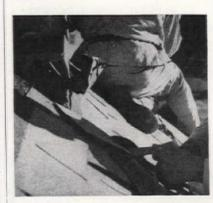
If old chimney flashing is not corroded, it can be pried up so that the new shingles can be cut to fit around chimney
