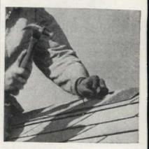
Shingles for cap should be nailed at corners. As there may be several additional layers of shingles at this point, it may be necessary to use longer nails for the cap than were required for rest of roof. Cap shingles should be overlapped to produce same amount of exposure as roof proper
