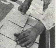
First course of shingles is laid over starter course. End of first shingle in this course should be cut off so that the cutouts will be centered over the tabs in the course below, Succeeding courses should be laid in a similar manner and in exact alignment
