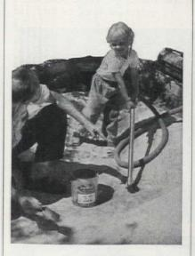
Portland-cement paints are applied to a dampened surface, but if a rubber base paint is used. the concrete should be bone dry. Just before the paint is applied, it is a good idea to give the pool a final sweeping. An ambitious moppet armed with a vacuum cleaner is a fine method of removing small bits of dirt and debris that get blown into the pool at the last minute
