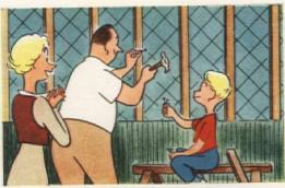
The dealer gave us simple instructions to follow. We started by nailing "filler" strips to make the wainscoting and upper wall even, so the final grainboard wall would be flush from ceiling to floor.
