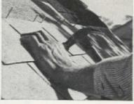
Each shingle should be secured by six 6d roofing nails driven through unexposed portion of shingle. Use one nail 1" in from each end, and two nails adjacent to each side of each cutout. These should be 1/2 above cutout, and 1" from midpoint. Be sure nails go into solid wood
