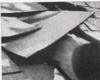
During warm weather, asphalt will be quite pliable, and the tab of a shingle nailed in place can be lifted up for joining up shingles in the lower course
