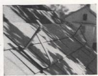
Adequate scaffolding is very important on a re-roofing job. Metal roof brackets can be installed easily and removed after the job is finished without leaving nail holes in the shingles
