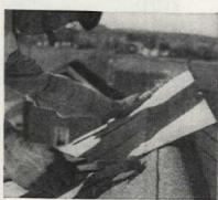
Shingles should extend far enough up on one side of roof so that the last course can be bent over the roof ridge and nailed to opposite side. Shingles applied to this side should also be bent over the ridge
