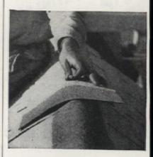
For ridge, cut each shingle into three equal parts with a knife or pair of tin snips. Place shingles over the ridge so that they run at right angles to regulation shingles. Be sure they are properly centered over the ridge and kept in proper alignment
