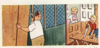
Then we nailed up planks of Gold Bond Gypsum Grainboard with a finish that looks just like knotty-pine and gives the walls a "fine antique" look. Planks are lightweight and easy to handle. You can saw and nail them as easily as wood. And they're fireproof!
