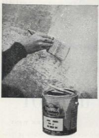
Ordinary oil paints are not suitable for concrete or masonry surfaces subject to constant moisture. It is best to use either cement paint or one of the rather new rubber-base masonry paints which will not be harmed by moisture or action of lime in the concrete. It is best to use an old brush to apply the paint, for the rough concrete will quickly wear down the bristles of a new brush, spoiling it for many future jobs
