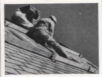
A length of 2 x 4, supported by four or more metal roof brackets, makes a good scaffolding and one which allows you to work the entire width of the roof without having to reposition the scaffolding
