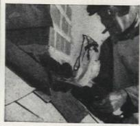
Strips of noncorrosive metal should be installed over the shingles to serve as base flashing. These are bent up so they run up under the cap flashing
