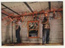
3 Radiators and registers gone! Coils of Bundyweld, shown before being fastened to ceiling, give ample warmth. Absence of dirt-catching radiators and dirt-spreading registers gives you freedom in furniture arrangement, provides many extra square feet of usable floor and wall space.
