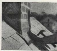
The cap flashing is now brought down to cover the base flashing, and nailed through shingles. Seams between flashing and shingles can be sealed with roofing cement
