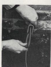
Pass ½ in. conduit through hole; fasten with lock nuts. Remove sod carefully, and dig trench for cable; then pass cable through conduit. Trench for cable should be from 6 to 12 in. deep
