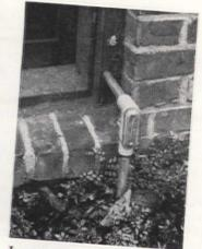
In some cases you will find that the conduit can be run through basement window frame. Hole should be drilled in frame, and caulking compound used to seal joint
