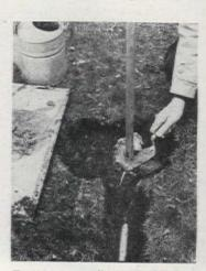
To support conduit, surround base with stones; then bond them with concrete. Allow the concrete to dry hard, and then replace dirt and sod
