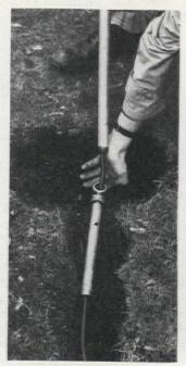
Stand for outlet box is made with two pieces of conduit and an elbow. Run wires through conduit and elbow pieces, and then assemble as shown
