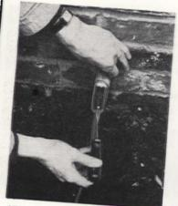
Allow a sufficient amount of cable on inside of basement to make a connection to an outlet box. Be sure circuit that you tap into is not overloaded. Replace plate on elbow
