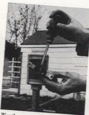
Weatherproof outlet box is attached to end of conduit; wires are fastened to receptacle. Connect other end of wires to junction box in basement THE AMERICAN HOME, JULY, 1953
