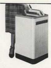
SMALL WASHING MACHINE takes up little space, washes six pounds of clothes in four minutes. Wringer folds into the aluminum tub, flat top covers it. AC-DC washer is 30" high; top, 161/2" x 171/2". \$120. Hoover Co., N. Canton, Ohio
