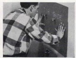
2. Reverse cardboard. With penknife, cut holes indicated by chalk. Place template over fittings to double check
