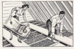
2 POUR IT, LEVEL IT, LEAVE IT! You'll be amazed how quickly you can do the entire job. Pour ZONOLITE directly from the bag between attic joists and sidewall studs. Flows freely and snugly around pipes, wiring and braces. Just pour and level . . . no muss, no fuss!
