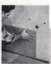
17. Apply base and lavatory panels same way as tub panels. Remember to apply mastic to within 1/2 in. of edges or holes
