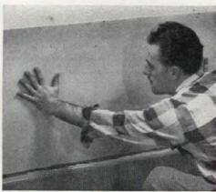
8. Scorings allow for expansion of mastic when pressure is applied in setting. Place panel on match covers. Press against wall
