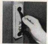
If your storm door is set so deeply that your knuckles scrape on the jamb when you grasp the handle, cut an "angle-block" from scrap lumber and fit it between the edge of the door and the handle
