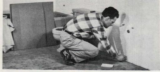
Three simple steps before ordering glass: measure tub wall; measure baseboard; make cardboard templates of plumbing outlets. Dealer supplies mastic and glass cut to size, with holes for fixtures
