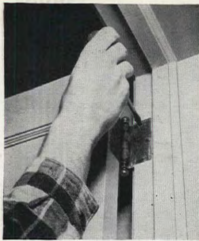
1. If door sticks, check hinges for loose screws. If screws won't hold, glue wood plugs in holes, or fill with plastic wood, let dry thoroughly
