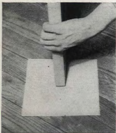
6. If door binds on bottom, slip medium-coarse sandpaper under it, swing door across it several times
