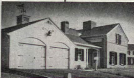
NO. 25 (see Oct. '53) Two-story Georgian with living room, dining room, kitchen, utility room, two bedrooms, and bath downstairs; two bedrooms and bath above; large closets throughout plus two-car garage and porch
