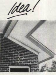
How to get adequate ventilation in the attic crawl space can be a very serious problem to homeowners. One excellent solution is to install perforated hardboard on the soffits— 1/4" material is usually sufficient. To prevent insects entering the crawl space, tack screening to the upper side of hardboard before installation
