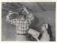
Start by nailing wood strips to your ceiling. Then attach clever Upson Floating Fasteners to these strips. Fastener prongs firmly grip Upson Ceilings from behind but don't show through. No visible nailholes.
