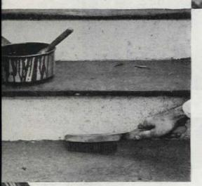
TEPS AND PORCHES lose their surface paint to gritty shoes in slushy weather. Come spring, they may be down to bare wood, and require a new protective coat. Be sure to clean out all dirt and loose paint with a wire brush or scraper before painting. Then a good coat of primer should be applied and allowed to dry, followed by two coats of the best floor and deck enamel you can buy.
