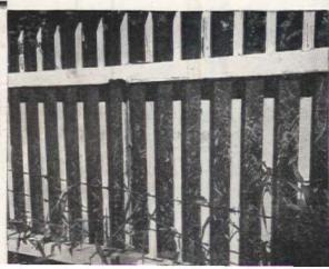
Snow drifts can cause individual pickets to break or may have pushed the whole fence over. Frost heave can disturb supporting posts, and moisture may have caused rot to start at the base of the posts. Investigate for loose pickets that ice may have forced away from the cross members, and see how paint has weathered winter storms.
