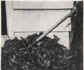
ROUND LEVEL tends to build up over the years, and though this is not only a result of winter weather, it is a good thing to check. To keep out dampness and insects, there should be a clearance of 18 in. from the ground to the top of foundations. If distance is less, dig down to proper level, saving sod for reuse. Make sure that your new grading slopes away from the house or you may get a damp basement.
