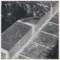
Here's a mowing strip of bricks and a single row of bricks at right angles to it (both laid in cement) separate the lawn from the flower border or garden walk
