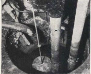
OUMP PUMP had better be in prime condition when the spring rains set in. A wire brush comes in handy for getting scum and debris out of the pit. See that the pump operates freely and, if necessary, lubricate the motor bearings. While you're "down cellar," check the walls and floor to see if any new cracks have developed which may let in the heavy spring rains.
