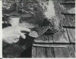
ORTAR often gets chipped and cracked out from between stones and bricks by ice and snow. If a small hole allows water to enter and freeze, the hole becomes larger, and the pointing is cracked out. Eventually, the masonry itself may crack or be pushed out of line by the ice that forms between it. Cure is to chip out loose pointing and refill cracks.
