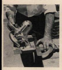
Calibrated quadrant on front of saw makes accurate bevel-cutting simple. Angles varying from 0° to 45° can be set by loosening wing nut, tilting shoe to proper angle, and retightening the nut securely
