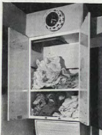
Standard kitchen cabinet at left is receiving end of laundry chute from second floor. One at right, over range, exhausts cooking odors: small motor and deep-pitch rubber blade are mounted in section of galvanized stove pipe running through cabinet, then under soffit to outside wall
