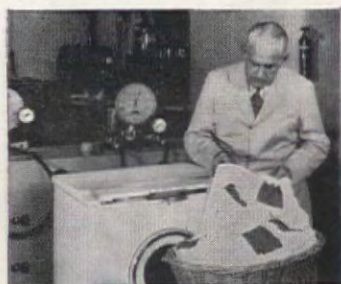
ATOMIC TESTS used Geiger Counter to accurately measure amount of dirt removed from cloth impregnated with radioactive soil.
