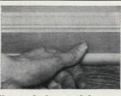
You can also locate studs by finding where baseboard is nailed to wall. Studs usually run in vertical line above nails
