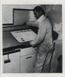
Attach sink to counter before mounting on base cabinets. All counters are screwed onto bases from below. Holes are provided for screws in bases. Connect plumbing—and job is finished!
