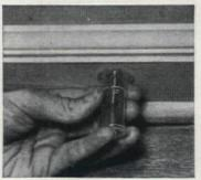
A commercial stud finder or dime store compass will point out nails in studs. Slide either one along baseboard. Needle deflects to indicate nail (stud location)
