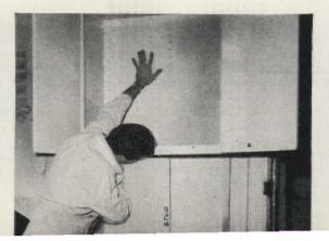
On stud walls, drill holes through cabinet back, on line with previously located studs. Use at least four 2-inch screws to fasten cabinets to studs. If this can't be done (due to location of the studs), use toggle bolts through wall for extra support
