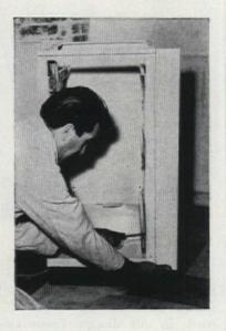
Though cabinets come in a great variety of widths, they can rarely be planned exactly to fill all the available space. Use filler strips (available in different widths) at one or both ends of the cabinets to give a continuous front. Cut the fillers to size, if necessary, and bolt to the cabinets before attaching cabinets to the walls. The fillers need not be attached directly to wall but should fit snugly to keep dirt from getting behind cabinets
