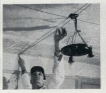
2. Lower ceiling fixtures. Locate halfway points at each end of room and snap chalk line between them. Snap second line across center of first line at right angles to it
