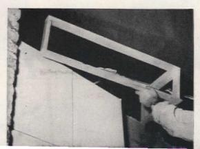
Build soffit into space, board by board, making sure that all faces are plumb, and that frame goes all around the opening. Nail to ceiling and wall with cut nails, and cover with wallboard, flush with cabinet front MORE ON PAGE 132
