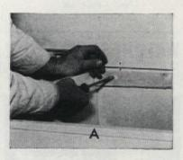
Attach sink front to adjacent cabinets. Then attach a strip of 1 x 2 to wall at rear as support for back of sink top. Your dealer will custom-build counter tops to fit your kitchen, or you can save money by using ready-made top sections
