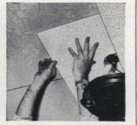
5. To fit around fixtures, cut tile with keyhole saw. Check each tile to see that it is flush with neighbors. If tile is set too deep, remove it, add adhesive, and remount
