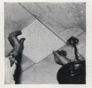
4. Start tiles where chalk lines cross. Press tile against ceiling  $\frac{1}{2}$ " from final location and slide in and out of place at least once to insure a good adhesive bond
