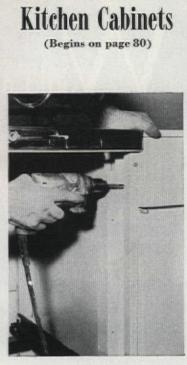
Both base and wall cabinets should be bolted together in groups before attaching them to walls. Otherwise, since few walls are absolutely straight, you may have difficulty in keeping fronts aligned. If holes are not provided, drill them, making sure to align tops and fronts before drilling. If bolts are not provided, use 10-24 x 3/8-in. round head bolts and a number 9 drill to make the right size holes, then cabinets won't slip out of alignment
