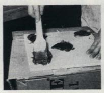
3. An inch from each corner of back of tile, apply walnut-sized blob of adhesive. If adhesive is closer to edge, it may squeeze out between seams during installation
