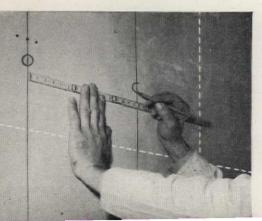
Place wall cabinet in position on wall, using strip of lumber as support. On solid walls, mark wall through holes in cabinet back. Remove cabinet, drill holes in wall with carbide drill. Insert wood plugs or lead anchors for supporting screws
