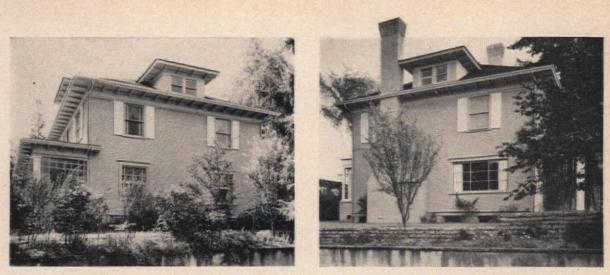
They added a well-proportioned chimney for the new living-room fireplace, and a large window in the dining room. Now there's a neat retaining wall and well-placed planting instead of the meaningless, overgrown, untidy assortment
