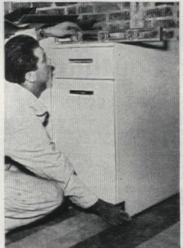
Before attaching base cabinets to walls by methods previously described, level cabinet with wooden wedges between cabinet and floor. Drill for studs or wall plugs and attach as described on page 80. Add cove base later to hide wedges
