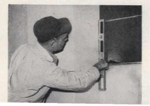
In most kitchens, it is inconvenient to use cabinets that go all the way to ceiling. Space left between top of cabinet and ceiling should be filled with a soffit. This can be built to fit space, out of  $1 \ge 2$ and  $2 \ge 4$  lumber as shown here
