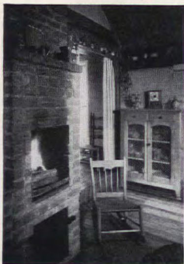
Kitchen fireplace sports a woodbox below, with firebox built at non-stoop level. Brick wall extends to form a convenient work counter
