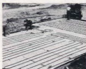
Installation of radiant heating Coils for typical modern home
