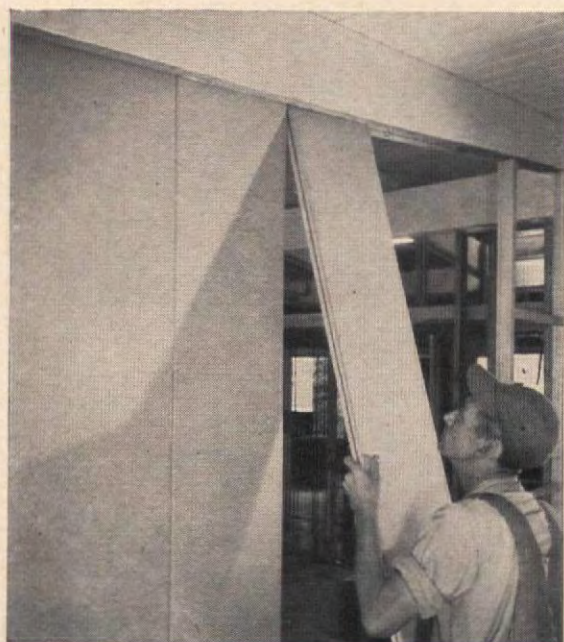
NO STUDS ARE NEEDED in this new method of building interior partitions. Baxbord panels have tongue and groove edges on long sides, slip into slot in rafter, are secured to floor by wood runners on each side of wall
