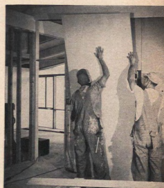
FINAL WALL IS 2 1/4" THICK. Basic panel comprises two Sheetrock panels laminated at mill. On job, a 3/8" thick, 4' wide panel is applied to both sides of wall
