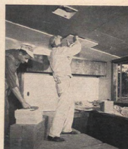
ACOUSTICAL TILE ON CEILING of kitchen effectively muffles clatter of clean up and noise of dishwasher's cycles
