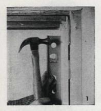
1. Measure the rough opening, then see if it is square, level, and plumb. Cut track, top and side door frames to fit opening. Assemble and paint frame, then slip it into place. If necessary, use small blocks to square up the framing. Then nail the assembled frame into position.
