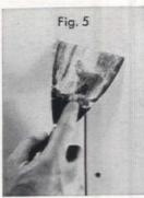
sions with a smooth coat of cement and let the cement dry for 24 hours. Then apply a second coat to the joints and nail heads, feathering it out on each side for several inches. The next day, apply a third coat, and feather this final layer out about eight inches on each side of the joints. Give the
