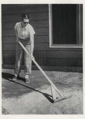
Then we spread and tamped down a 1" layer of sand on top of the crushed stone base. We checked the surface of sand for \(^1\)4" drop in each foot—same as slope of ground beneath. The sand gives bricks firm support.
