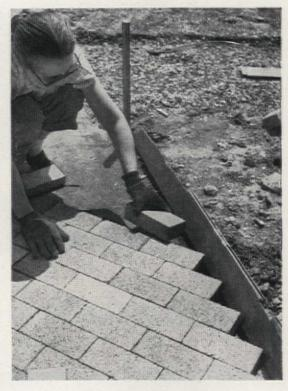
On the sand layer, we laid the bricks, leaving space of \(^1/\_4\)" to \(^1/\_2\)" between bricks. We used straight board to guide start of each row. With all bricks down, we swept sand over them, and dampened with garden hose.
