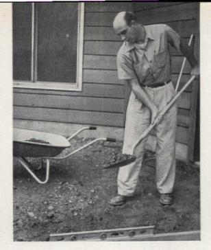
We did final grading ourselves. Terrace area had to be dug deep enough for bricks to come flush with level of lawn. For water runoff, we sloped terrace from the house, dropping \(^{1}\)4" for every foot of terrace width.
