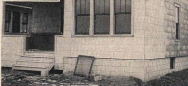
This owner built a full basement for added storage and a recreation room. He enclosed part of his front porch to lengthen the living room. And then he finished the outside walls with asbestos-cement shingles—a durable exterior that will require little upkeep for years of service.
