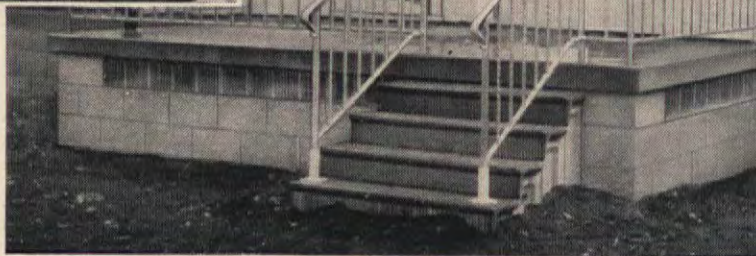
The basement which was added to this house was extended to the front and roofed over with a cast-in-place concrete slab. This became the floor of the pleasant new front porch shown in the large photo above.
