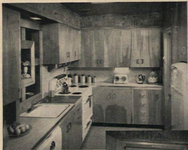
New birch kitchen takes up same space as old kitchen, but plan now allows better storage space, and over-all efficiency. Living-dining area beyond pass-through.
