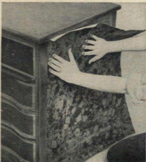
6. Brush paste onto back of wallpaper panels, one at a time. Cover every inch of paper smoothly, evenly. Smooth paper onto desk with hands.
