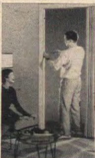
Screw clips to door jamb
