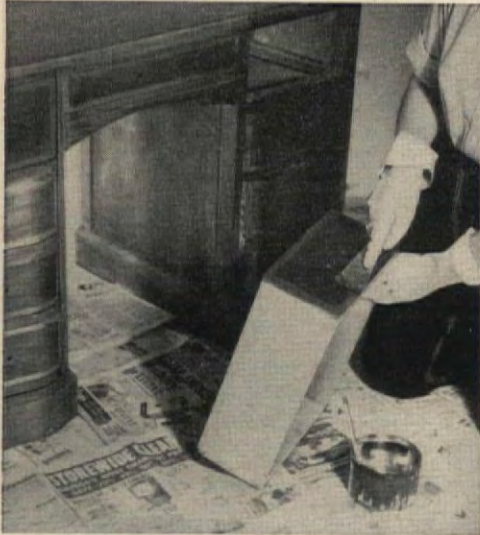
1. Spread papers on floor. Remove hardware. Apply paint remover with brush to remove finish. Scrape blistered finish off with putty knife.
