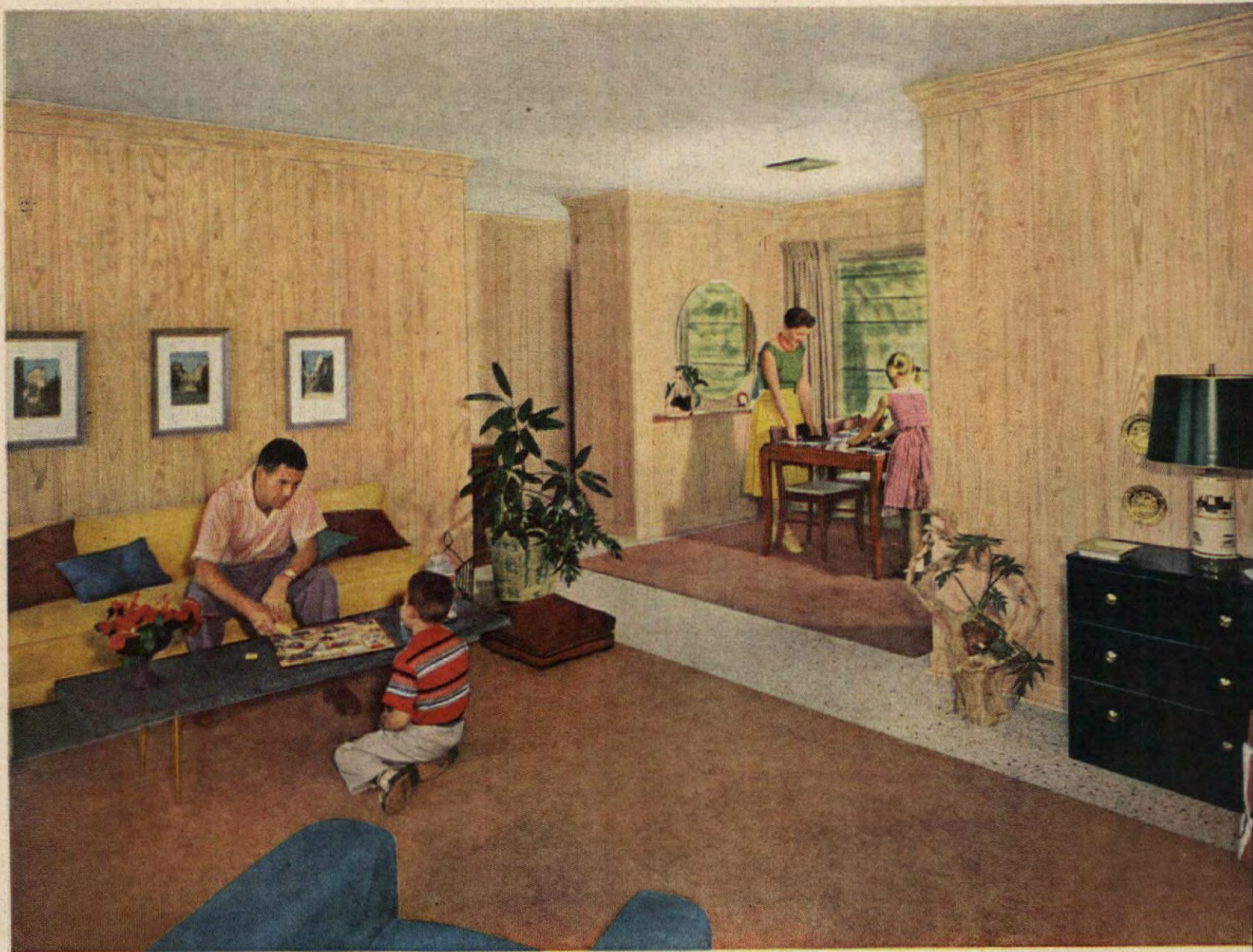
Recreation room, living room, and dining area, as well as the front entry and hallway, are paneled in handsome cypress, alternating 6" and 8" V-joint boards. The wood was given a coat of sealer and a thinned-down wash of pottery white paint to produce bleached effect.
