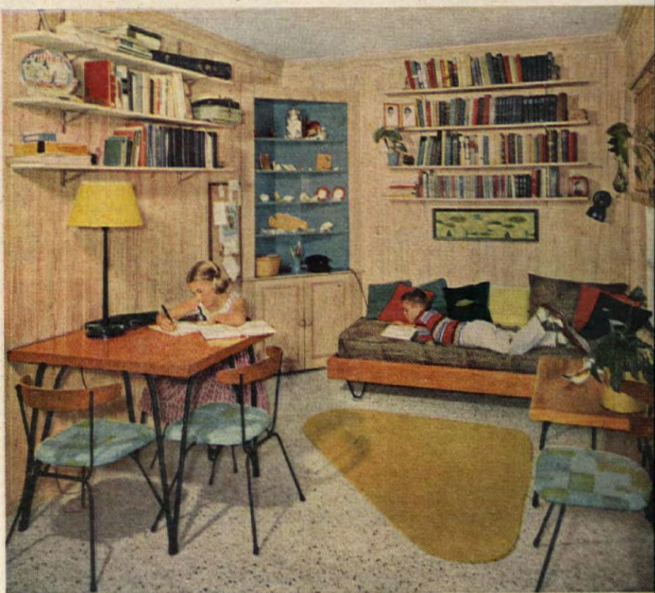
Recreation room, living room, and dining area, as well as the front entry and hallway, are paneled in handsome cypress, alternating 6" and 8" V-joint boards. The wood was given a coat of sealer and a thinned-down wash of pottery white paint to produce bleached effect.
