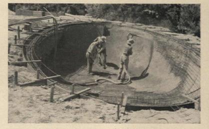
BLOWING CONCRETE under high pressure over, around steel reinforcing mesh in excavation makes "gunite" pool. No forms needed to hold concrete.
