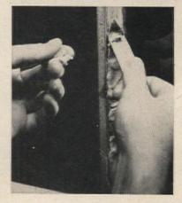
6. Roll putty into strips the size of a pencil. Lay these strips all around the outside edge of glass, over the glazier's points. This putty should be put on in a small enough quantity so it will not be visible to you from inside the house. Use putty knife (or can-opener) to smooth at correct angle.
