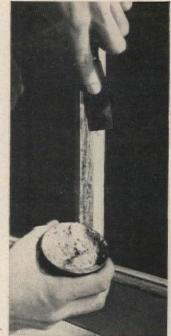
4. Before you put in glass, use a putty knife to apply a 1/16" layer of putty over the linseed oil. The layer of putty helps cushion the glass against shock, helps keep out drafts and rain.
