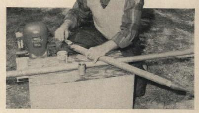
'Now you assemble your driving shaft: use well-point and lengths of pipe that are joined with pipe couplings. Ask well-equipment supplier for proper well-point to use in your kind of soil. In getting pipe sections ready to join together, he sure you spread pipe-joint compound on the threads; screw couplings tight to prevent leaks. PLEASE TURN THE PAGE
