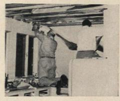
Mr. Mason staples reflective insulation between ceiling joists in kitchen. Next: furring, acoustic tile.
