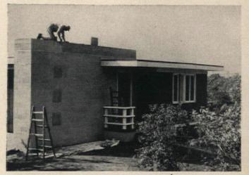
Almost done: concrete cap is troweled over the top of the chimney to keep water out of chimney blocks.
