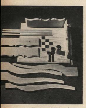
Cut apron and legs from 1" birch stock, cut top from  $\frac{3}{4}$ " plywood. Checkerboard is made of  $2\frac{1}{8}$ "-sq. hardwood veneers (in hobby kit). Lay squares in straight lines, as in drawings.
