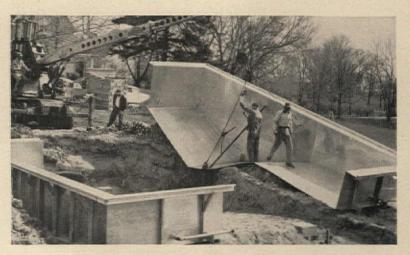
METAL POOLS are popular. This aluminum model arrives in two lengthwise sections ready to fit into the ground. Notice pipe connections are installed.
