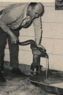
Use a sand-mix, packaged cement to make a slab for pump. While slab is still wet, insert bolts to fit holes in base of pump. A form for concrete base is easy to make with 6"wide wood scraps held in place with small stakes. Use a T-fitting to connect well to pump. Connect motor to electric outlet.
