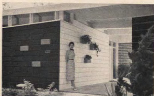
Conventional block with deeply raked horizontal joints
