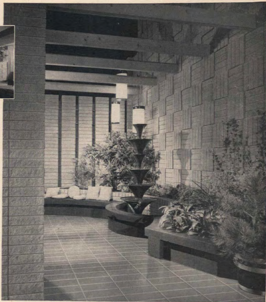
Rugged split block combined with smooth-faced block laid in a basket weave pattern
