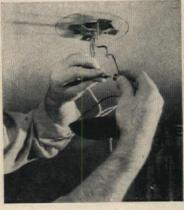
Place your new fixture over the mounting, first making sure that no bare wire protrudes under the connectors.
