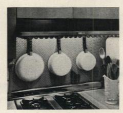
This new hood with its own pushbutton control hidden in the name plate, turns on the blower fan, concealed in the cabinets above, and turns on the light over the range.
