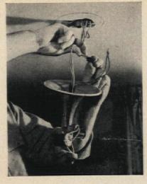
Before unfastening old fixture turn off current at master switch to prevent any chance of electrical shock. Then remove any glass parts and bulbs and unscrew fixture from the ceiling mounting. Disconnect fixture wires from wires coming through ceiling by untwisting solderless slip connectors that join the wires together. Soldered wires will have to be snipped in order for you to be able to separate them.
