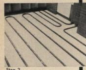
Install radiant panel or grid of steel pipe and connect with existing hot water heating system.
