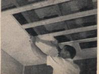
My lumber-yard bill came to roughly \$200. Installing studs for the new walls, firring strips for wallboard and the wallboard itself were the quickest and easiest jobs. The most time-consuming were the finishing touches . . . laying the tile, taping mouldings and trim, paneling and rubbing the tongue-and-groove V-joint redwood. We wanted a professional-looking job and brother, that kind of job takes time!
