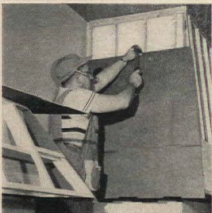
HARDBOARD WAS CUT to look like slate; extended from "roof top" to ceiling.
