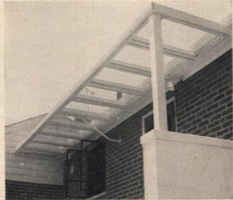
1. BUILD AN EGG-CRATE OVERHANG as permanent part of the house, made of 2x4's. Pipe truss support in center reduces chance of sag. Space 2x4's on 2-ft. centers. Screen individually.
