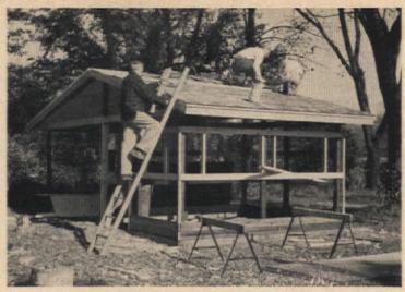
3. ROOF IS MADE UP of 1x8'' sheathing nailed at right angles to rafters. Over sheathing go roofing felt and asphalt shingles. 1x2'' trim board is nailed to eave edge of roof sheathing.
