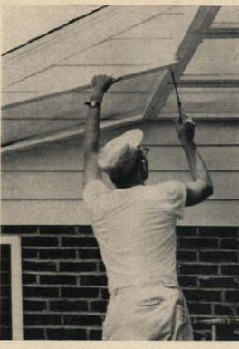
5. AFTER FITTING the screens on the egg-crate overhang, the portable roof screens go up. Screw screens to plate and to the edge of the overhang. When all roof screens are installed, the door frame and corner posts will be sturdy and quite rigid. Note: It will be necessary to make the double or single door frame, leading out from terrace, of 2x4 framing to accommodate the thickness and width of the door.
