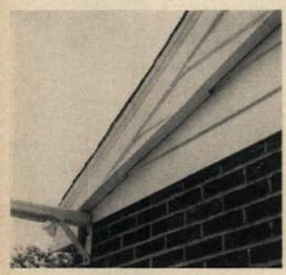
4. SET PLATE in place. Scribe starter strip to siding to insure tight fit, study photograph carefully. Door posts and corner posts are fitted to plate with bases pinned to holes in the terrace edge. This terrace is only bounded on two sides, so only one corner post is required. Free end of the plate was fastened to a bracket fitted to the garage wall.
