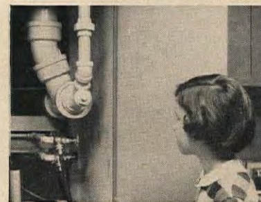
PIPES DISAPPEARED behind furred-out walls, but essential connections are still accessible whenever needed.
