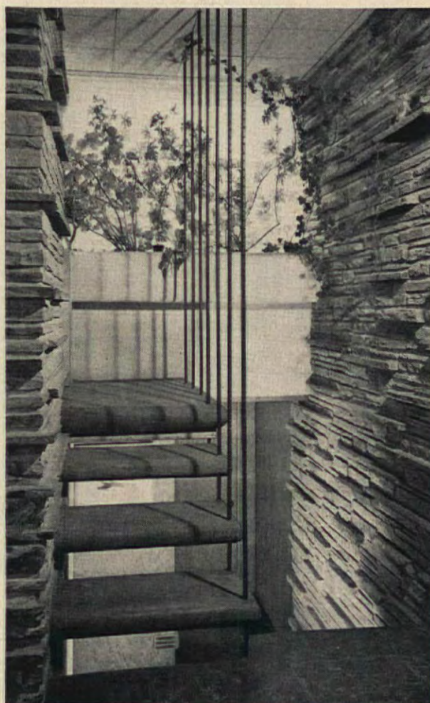
A LIGHT LOOK and a sturdy stairway can be had with these steel supports and molded cement steps. The see-through risers for a contemporary touch are as attractive as they are functional.
