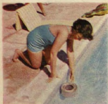
SURFACE SKIMMERS catch floating dirt, keep pool water clear.
