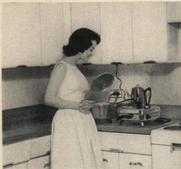
Appliances are plugged into outlets in hostess' kitchen to reheat before taking them outdoors. Saucepan and skillet use a double wall outlet, while the coffeemaker is plugged into an under-cabinet outlet on another circuit.
