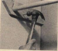
You can make shelf supports for your closets that will do double duty by sawing out a groove in the support to hold the clothes pole.
