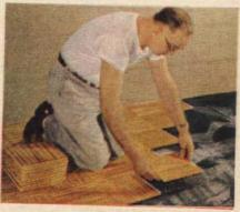
Easy to lay—Bruce Blocks may be installed with an adhesive over any smooth surface or nailed to a wood subfloor or old floor.
