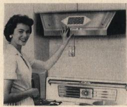
NO OUTSIDE VENTS are required for a range hood that attaches to wall and plugs into any 110-volt AC outlet. It dissipates grease, smoke, and odors electronically; purifies air, and then recirculates it. From \$79.95 to \$109.95. Puritron Co., New Haven, Conn.
