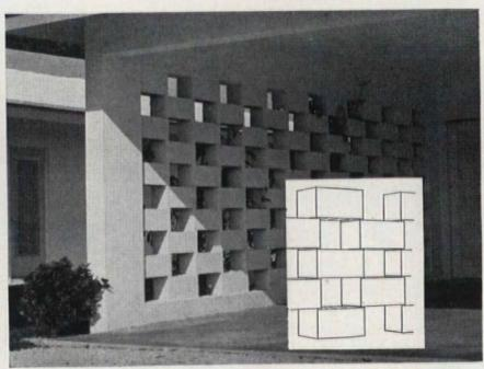
**Double corner blocks** stand here in a pattern as old as children's blocks, and just as satisfying. Excellent for a windbreak, or for the end wall in a carport. Support must be provided for end rows.
