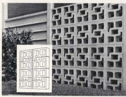
Corner blocks, like the chimney blocks shown at left, present an intricate design when placed on their sides. Stacked corner-up. corner-down, the resulting grille seems modeled and hand-crafted.
