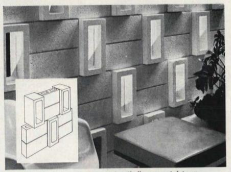
Standard single-core blocks are set vertically, core out, between pairs of stacked partition blocks. Adjustment of the projection of the "shadow boxes," and of row over row, calls for precision.
