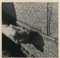
Mortar courses must be "tooled" to make them firm and water-resistant. This is true even when the joints are to be kept flush. The tool shown is the simplest; there are also tools to produce a  $\lor$  or concave joint.
