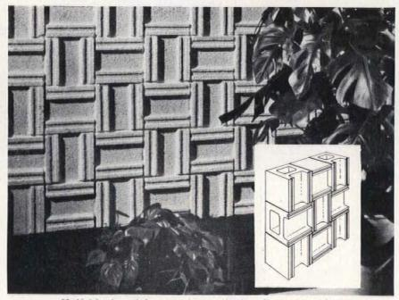
Half blocks with stretcher ends describe a strong basket-weave pattern. The simple alternating of the blocks, vertically, then horizontally, gives a light look to an otherwise heavy, solid wall. SEE PAGE 72 FOR HOW TO'S
