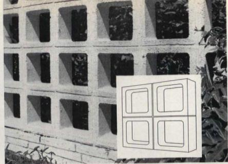
Column blocks stack up to create a large-scale design of great simplicity and strength. Best for a broad area; fine for defining a lot line; primarily a grid to see through, so be sure it faces a good view.
