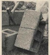
Cut blocks to size by scoring both faces with a cold chisel. Tap gently, slowly pulverizing along the line. When the line is scored, a sharp rap will break the block.
