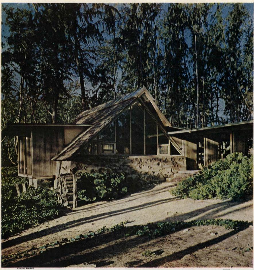
This vacation house is basically two tent-shaped structures, commonly called "A-frames," connected by a covered passageway or lanai. The larger structure serves as the living and indoor dining areas but can also double as sleeping quarters. Attached to it is a shedlike building that contains the kitchen and a bath-dressing room. The small structure contains two bedrooms as well as a bath.
