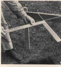
Use "batter boards," cord, and a framing square to lay out the trench for the footing. Corners at ends of wall must square with each other. Nails in the crosspieces that hold the cord should be at the precise line of the wall.
