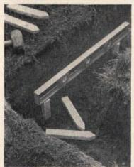
To insure that the footing is even, drive stakes into the bottom of the trench; use a level to make sure the tops of the stakes are all the same height.
