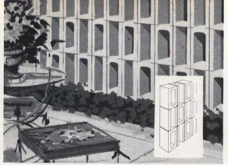
Lintel and single core blocks in checkerboard arrangement form an almost-solid wall with emphatic vertical lines. From the other side, the pattern is severe, so give a thought to that view, too.
