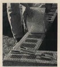
Use wire mesh reinforcing on the next-to-top course on all walls, and along every fourth course on high walls. Use vertical reinforcing rods if stronger support is required.
