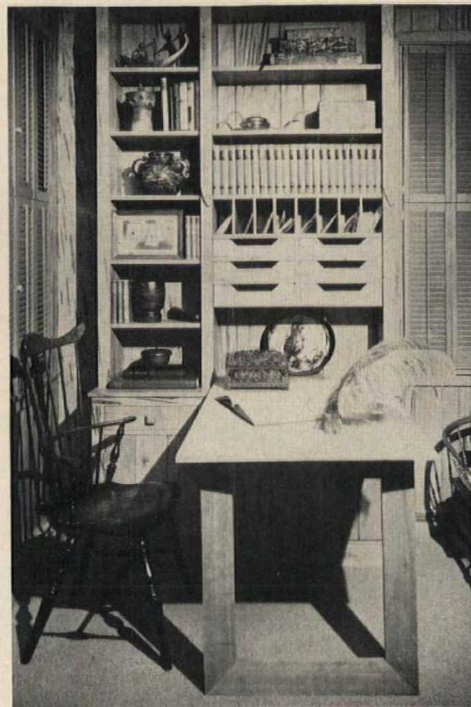
7. No room for a desk? Of course there is if you use this idea. Section of this built-in bookcase drops down to become a hard-surfaced desk and work area. Drawers, pigeonholes, and shelves are built in behind. Legs become frame on wall panel when it is closed. Home of Mr. and Mrs. R. C. Hensel.
