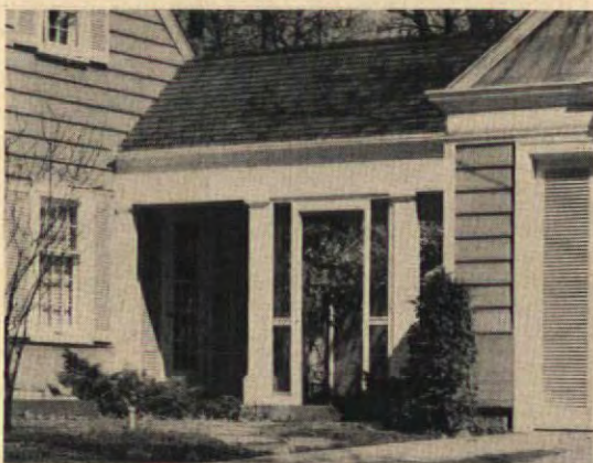
A natural framework for the much-needed family room was provided by the old breezeway. To get more space in the family room, the framing was extended toward the front of the house.
