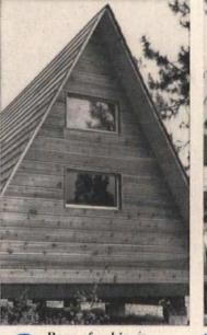
**6 Rear of cabin is** framed with 3x4" stock and covered with sheathing and cedar siding. Top window is for loft. **T Front of cabin** framing accommodates door and fixed or movable sashes. Siding used is 34" tongue and groove.
