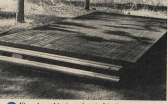
Floor for cabin is made out of 2x6" tongue-and-groove stock. Deck framework is covered with square edge 2x6s, set ¼" apart.
