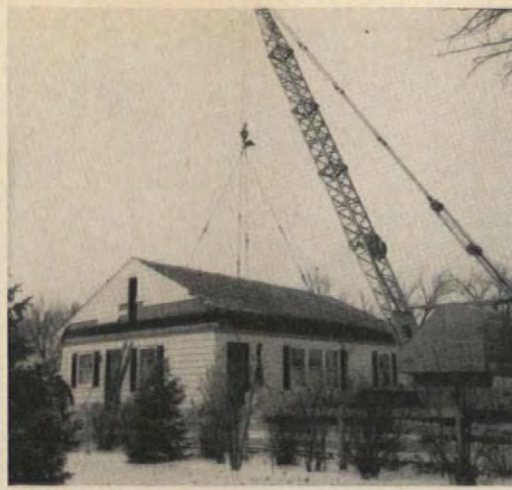
Second-story addition was accomplished by renting a crane with a 70' boom to lift the roof and replace it on the new addition.
