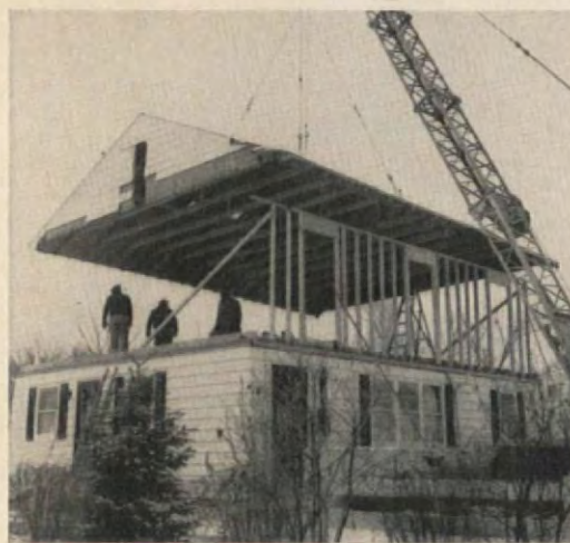
Three hours later the crane lowered the roof onto the side walls and it fitted perfectly. The rental of the crane cost only $125.
