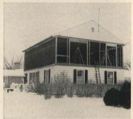
By nightfall the men had the sheathing up on three sides. They left one end open to bring in bathroom fixtures, covered it with plastic.
