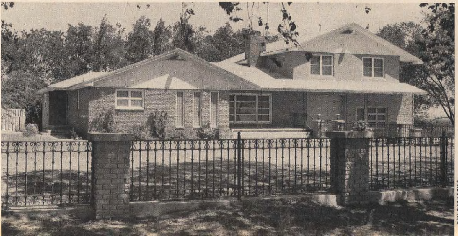
Amazing change included removal of outside stairway and the addition of one-story wing. Brick facing ties new and old together.
