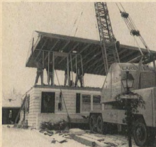
Workmen steadied roof with guy ropes. Meanwhile carpenters tilted up the side walls and a bricklayer extended the chimney.
