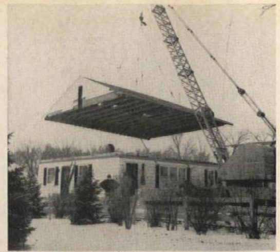
The crane hooked on at 10 A.M. and lifted the roof ten feet. Side walls were assembled and ready on the attic floor before crane arrived.
