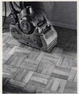
Sanding with an electric drum sander is best done by moving in an overlapping pattern until you cover the entire area. To leave the floor burnished and absolutely smooth, five different sanding steps are needed from the heavy duty sandpapering to the superfine cut sandpapering. Be sure to remove all the sediment from the sanding process before starting the next step.
