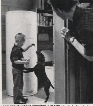
BECAUSE IT WORKS WITHOUT A FLAME, the Schultzes' electric water heater needs neither flue nor ventilation. This allowed the Schultzes to save valuable basement floor space by installing it in a windowless storage area.
