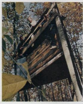
Architects of Kinne house used curtainwall construction to minimize framing and foundation work. Note how existing trees double as columns.
