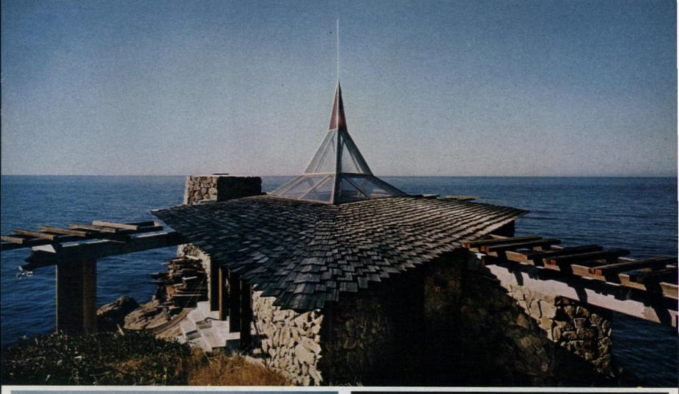
Wide-angle view shows large side arbors that are actually extensions of the main structural beams supporting the redwood-shake roof. Beams connect to base of cupola.
