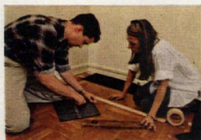
Carpet tile, held down with Scotch double-faced tape, cuts and fits easily.
