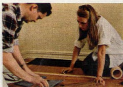
Carpet tile, held down with Scotch double-faced tape, cuts and fits easily.
