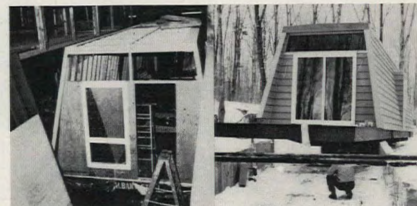
Factory assembly of each wing, or module, involved framing basic skeleton of trapezoidal wooden frames by machine-screwing to steel floor system.
