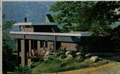
Exposed steel framework of Zimmerman house provides main support from above instead of underneath. "Cupola" on roof is master bedroom, with adjoining sun deck. Attached garage is seen in the foreground.
