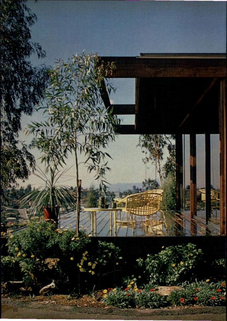
This Concept House, as it is called, costs \$13,500. Produced in a factory in Buena Park, California, it consists of two basic modules, each 12 by 40 feet, delivered by truck to this handsome hill-side site. Cost for cartage: \$1.40 a mile or 70 cents-a-mile per module, within 300 miles. Five other versions are available. Decks, for \$13,500 carport and landscaping custom-fit the house to its site. (continued)
