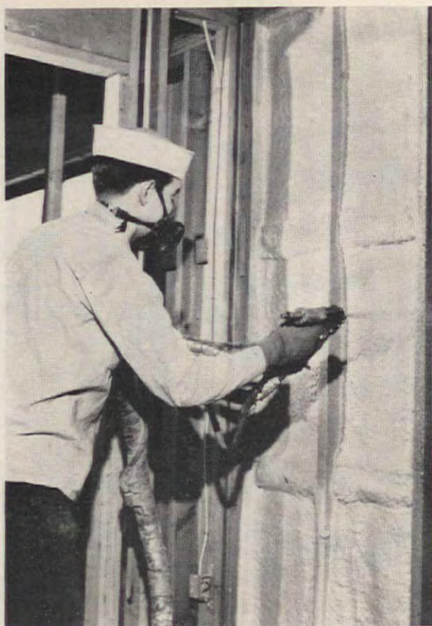
Urethane foam is applied as insulation and sealant in a new condominium at Heritage Village in Southbury, Conn.
