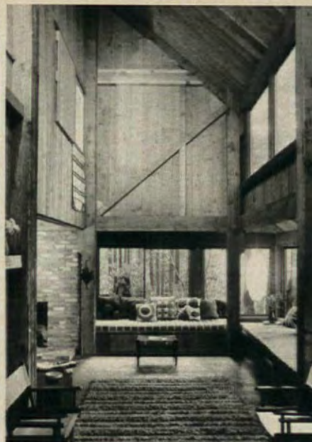
Ceiling soars 24 feet over living area (above). Diagonal bracing throughout the house is a California earthquake-protection requirement. Bedroom over dining area (above, right) faces living area through a barnlike "lookout."
