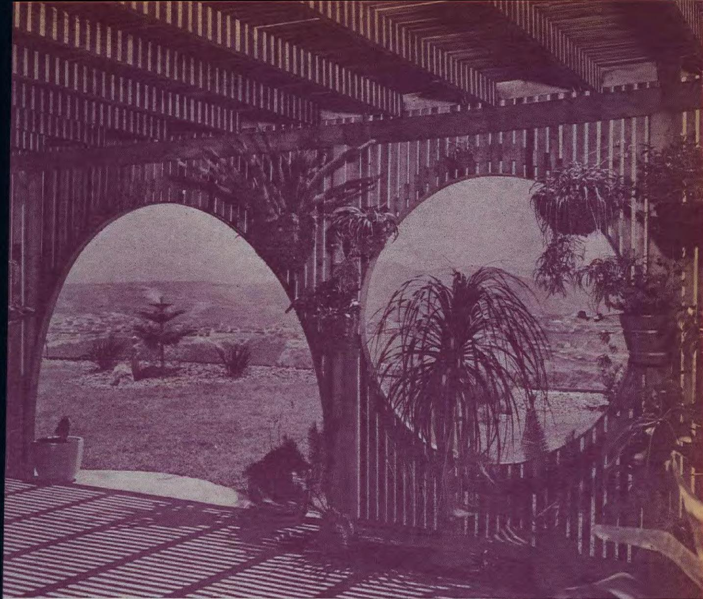
Trellis roofing rests on 4x4 posts anchored in concrete (below). Box frame of 2x6 beams set in cutouts on top of posts provides rigidity; intermediate rafters spaced at 2-foot intervals to support 1x2 slats are notched to fit over ledger strips at each side. Size and spacing of the post-and-beam framework must conform to your local codes.
