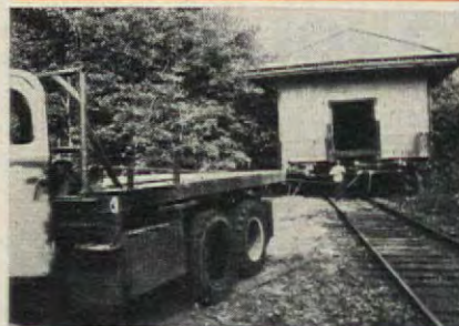
Station, hauled by truck, rumbles down tracks on dollies. It left tracks without mishap 400 yards from crossing.
