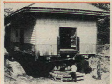
At bottom of prepared ramp extending from tracks to site are cement footings. Planks laid across stacks of pilings form smooth runway for dolly wheels.
