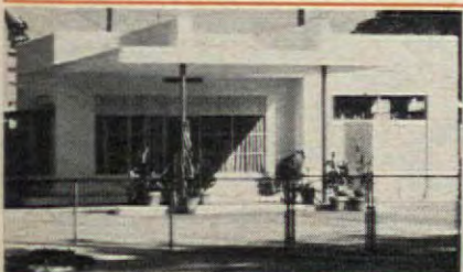
Remodeled into a spacious and handsome studio, Entrekin's old station now contains a library, workroom, bath, tiny kitchen area. Building was sanded and sprayed with pre-mixed concrete painted white.
