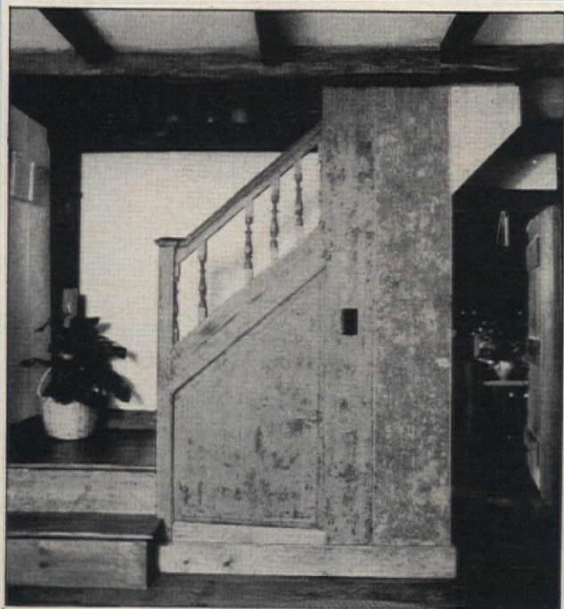
Antique staircase, stripped and shortened to keep kitchen doorway clear, replaced ladder leading to loft area that's now master bedroom.
