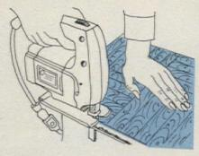
Elegant parquet floors are within reach of the do-it-yourselfer with the availability of new fcam-backed wood tiles that lay easily. Use a saber saw (above) to cut tiles to fit—at corners and walls.
