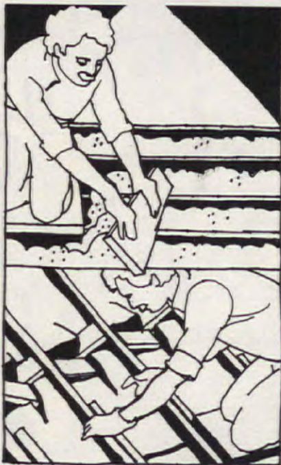
Use loose-fill or batts in attic floor
